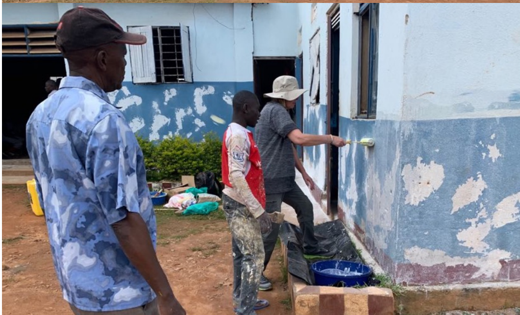
NEW PAINT JOB JACE PRIMARY SCHOOL IN THE SLUMS OF KAMPALA
